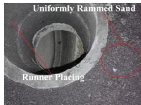
Fig. 16. Sand Ramming and Runner Placing
